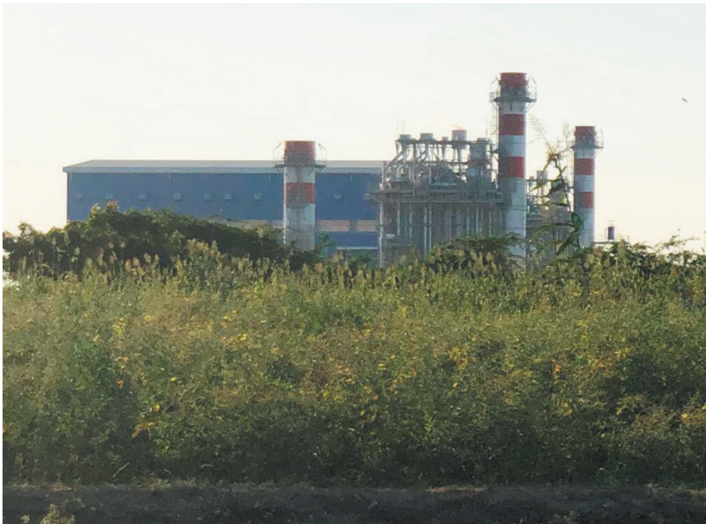
The Myingyan Gas power plant, Myanmar. Courtesy: Recourse
